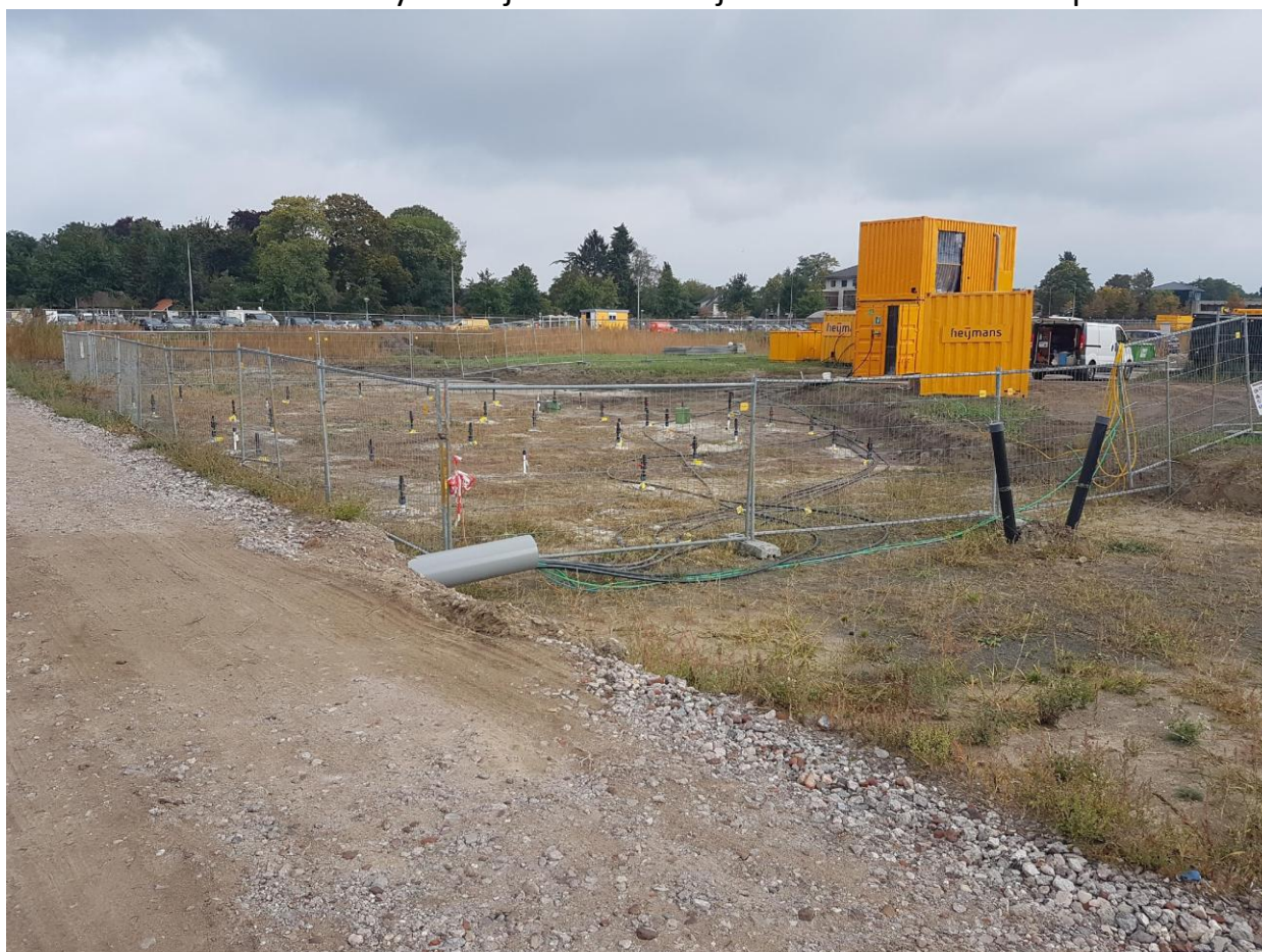
Overview injection filters in source zone
