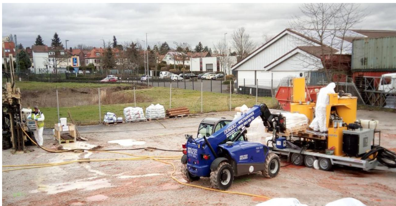
High pressure injection/fracturing/ and mixing equipment used for fracture-emplacement of persulfate-peroxide oxidant slurry into subsoils through direct push drill holes
