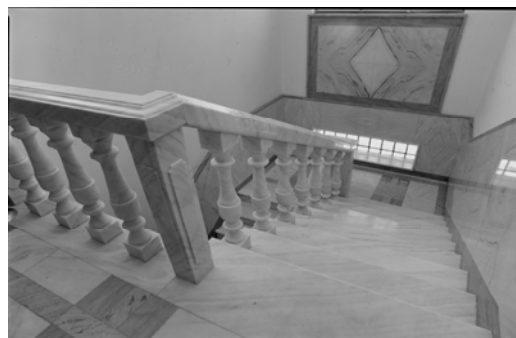
Fig. 3. Railing and stairs made of Ruschita marble.
