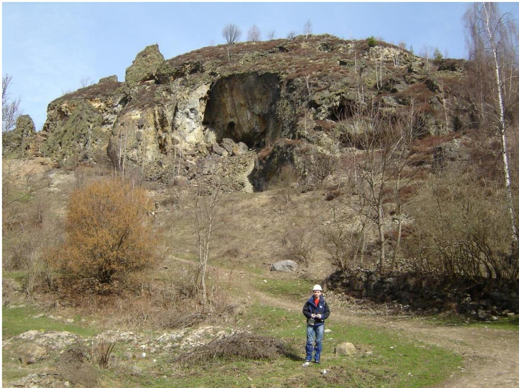
Fig. 3. The northern slope of Văidoaia massif with historical exploitation works exposed at the surface. The central opening is continuing underground towards north in its lower part forming a stope known by the locals as *Coranda Văidoaia*.
